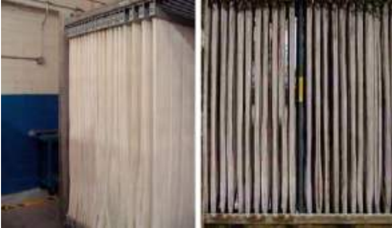
figure 7.4 - correct (left) & incorrect (right) slack adjustment
