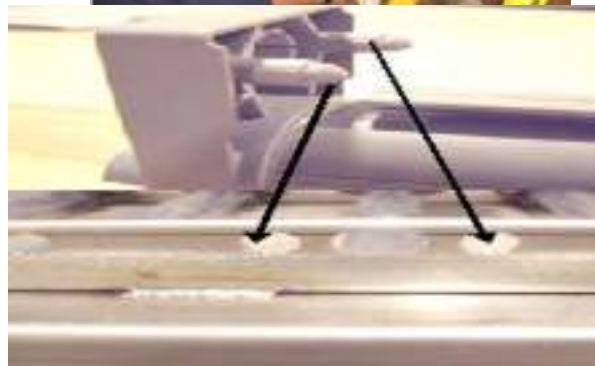
figure 5.26 - inserting the bottom header
