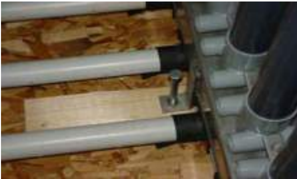
figure 7.14 - installing a bolt in the L-bracket tip Stagger the adjustment of the four bolts.
