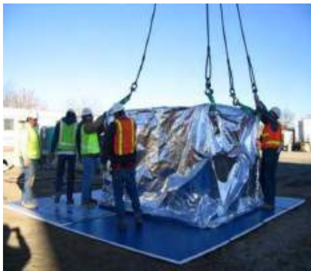
figure 5.9 - lifting cassette without a four-point lift frame & spreader bar
